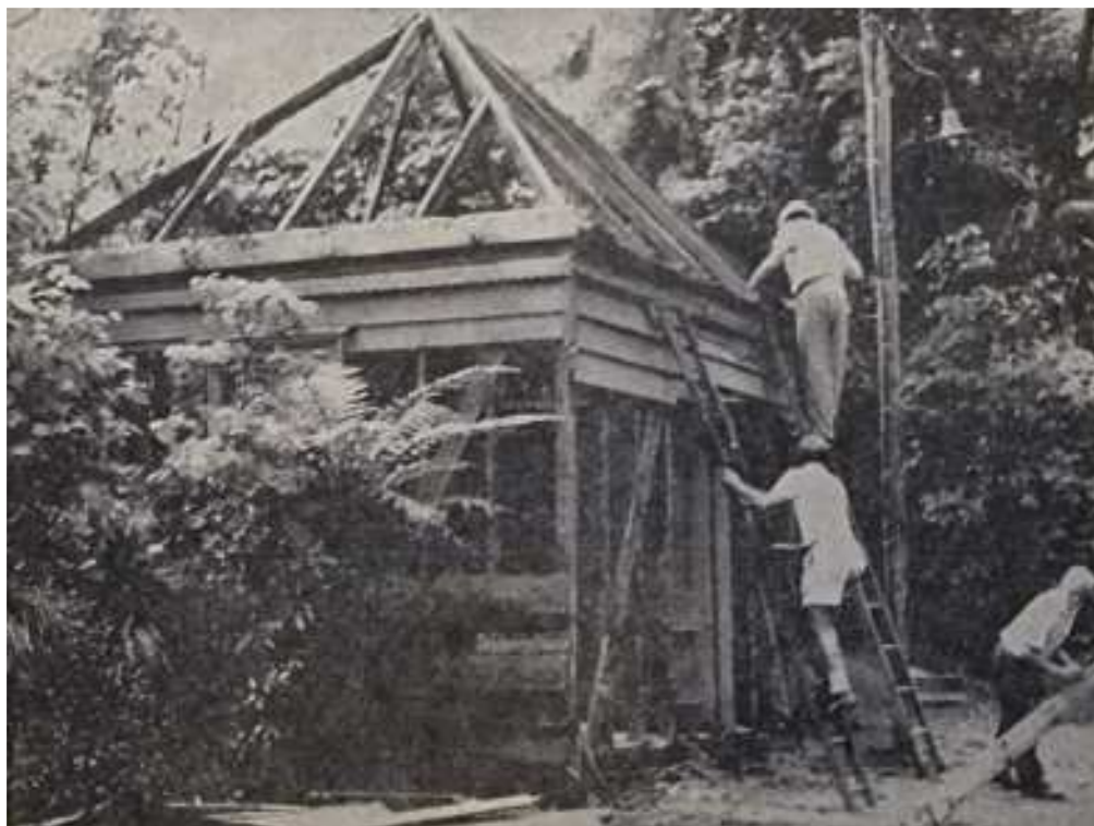
The old bathing shed being dismantled (Taranaki Herald, March 18, 1969)
