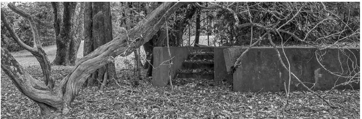
Below: The pavilion steps.
