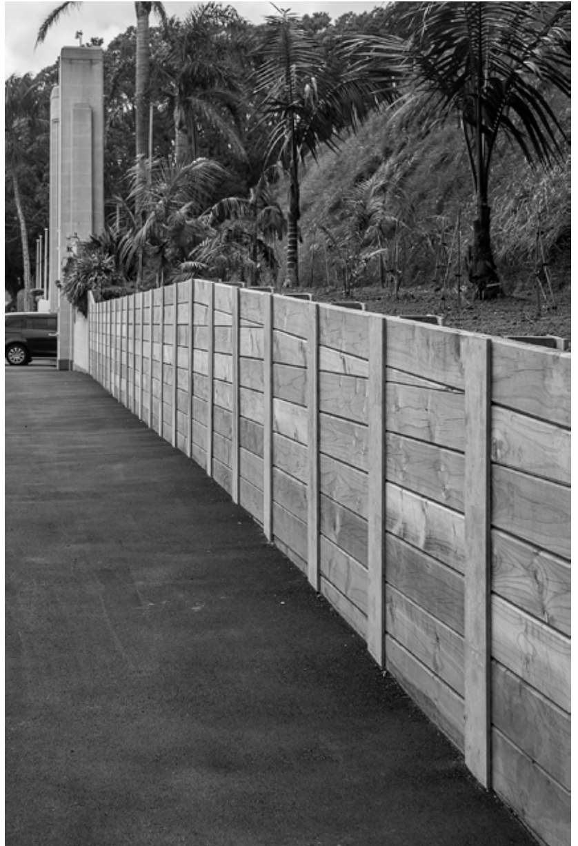
New Fillis Street wall.
